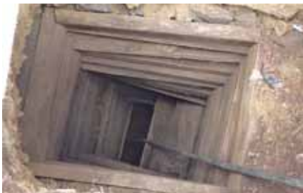
① Gold bearing rocks are extracted from a properly timbered mine shaft
