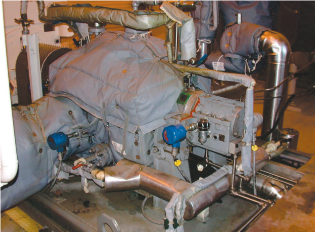
Figure 7. Heat Tracing and Blanket Insulation.
