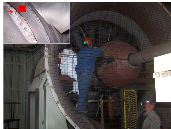
Figure 7 – Blade setting change
