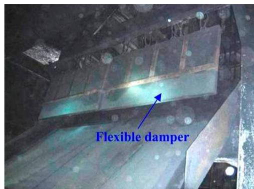
Figure 14. Flexible damper.
