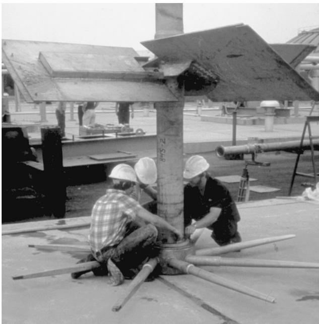
Figure 25. Full Scale Test (Installation) of 10 Ft Impeller and Rotating Air Sparge.
