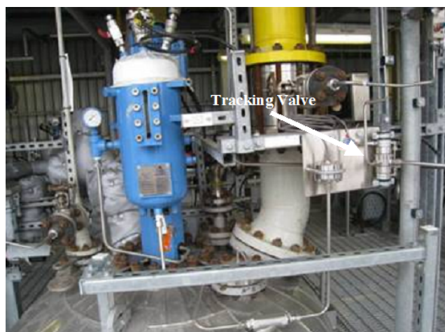
Figure 19. Tracking Valve Installation.
