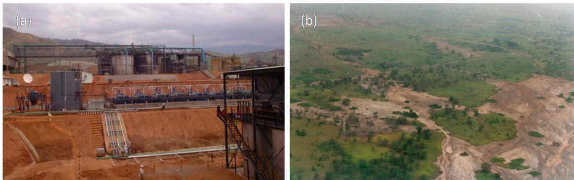
**Figure 7.** Bioleaching plant (a) for the processing of pyritic tailings (b) containing cobalt, copper, nickel and zinc. Photographs from D. Morin, Bureau de Recherches Géologiques et Minières (BRGM), reprinted with permission.
