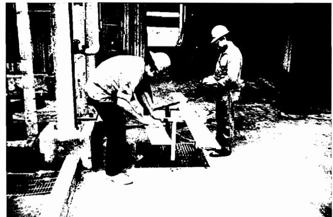
Figure 13. Three Coats of Paste Wax Must be Applied to all Grout Form Surfaces Coming in Contact with the Grout.
