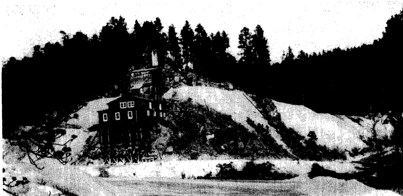
Heavy-Media separation plant and mine area, Keystone, S. D.
