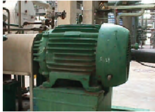
Figure 7. Totally Enclosed Fan-Cooled Motor (TEFC).
