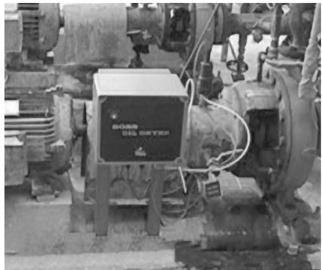
Figure 15. Automatic Oil Dryer in Use.
