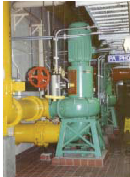
Figure 7. Vertical Frame Mounted (Casing Pressure Flange) Nonclog Pump.
