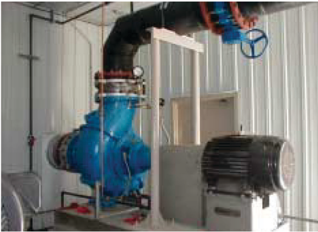
Figure 6. Horizontal Nonclog Pump.
