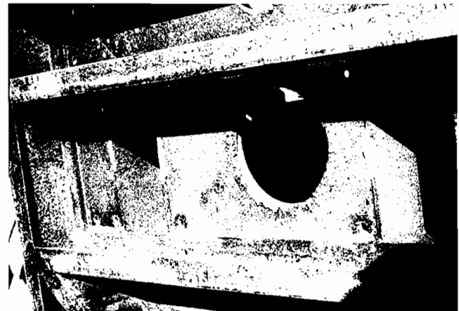
Figure 5. Underside View of a Fifth Edition Angle Type Baseplate.
