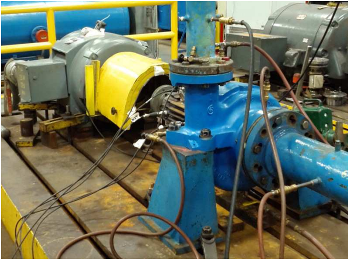
Figure 9a: Pump installed in the test loop
