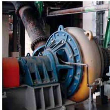
Left: Cover plate of a 550 MCR about to be installed at a copper plant
