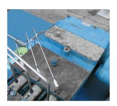
Fugitive emissions were virtually eliminated by this packing arrangement
