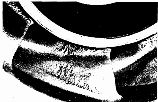
Figure 1. Typical Cavitation Damaged Impeller.
