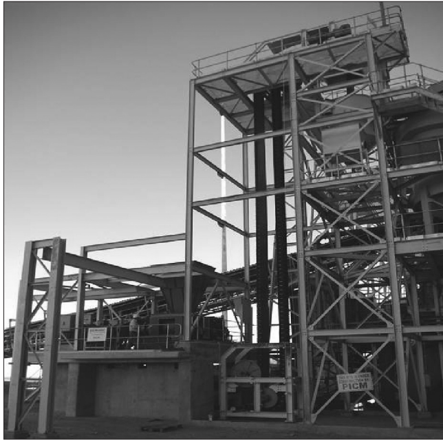
Figure 9. Northam UG2 Plant Polycom 09/06-0
