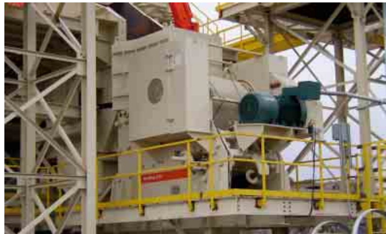
A C145 during the installation phase at a new primary crushing plant.
