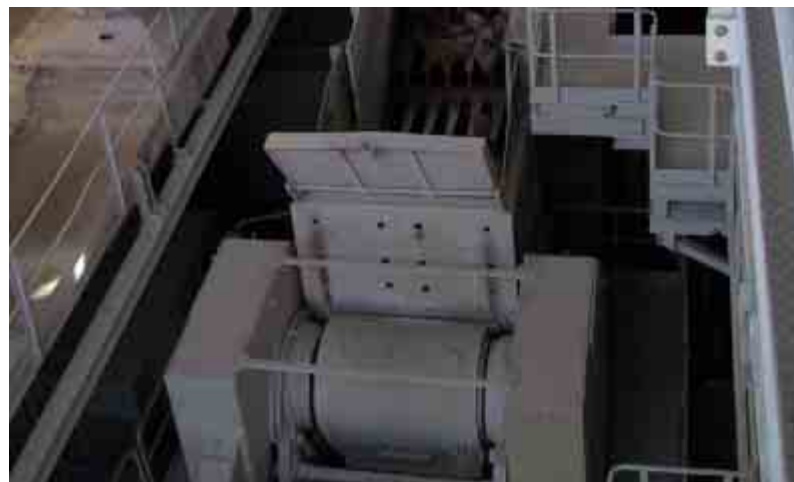
A C200 after replacement of a double toggle jaw crusher. Plant capacity was increased without having to modify the foundations.
