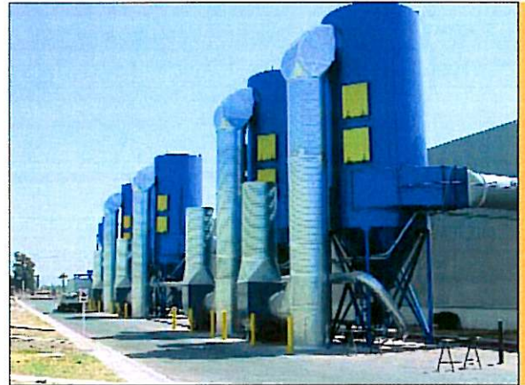
484RF four RF collectors on wood dust
