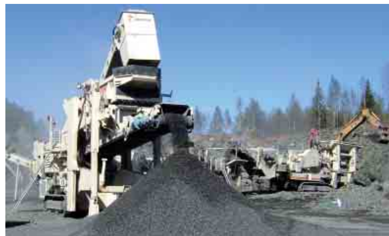
Three stage crushing and screening process with the Lokotrack LT110, LT300GP and LT300GPB.
