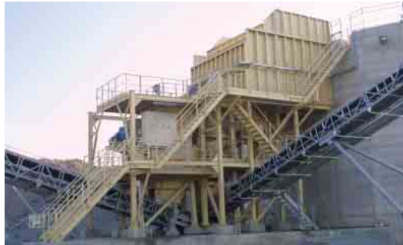
A C125 during the installation phase at a new primary crushing plant.
