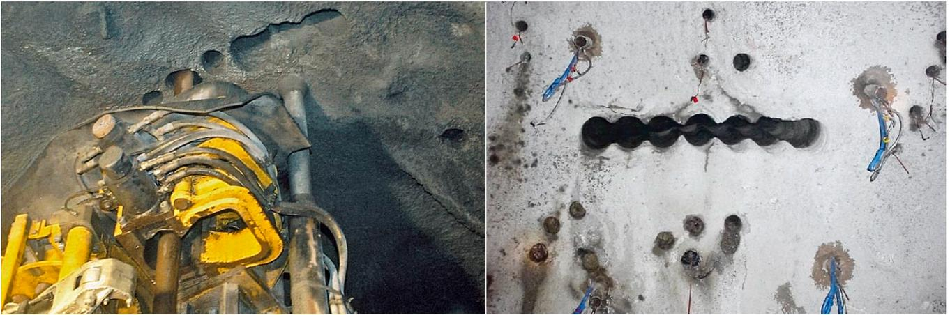
Slot drilling at Ferbasa: The Simba M6 C in action and, (right), the perfectly finished row of holes.
