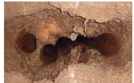
Sufficient expansion space is created for production blast holes to follow.
